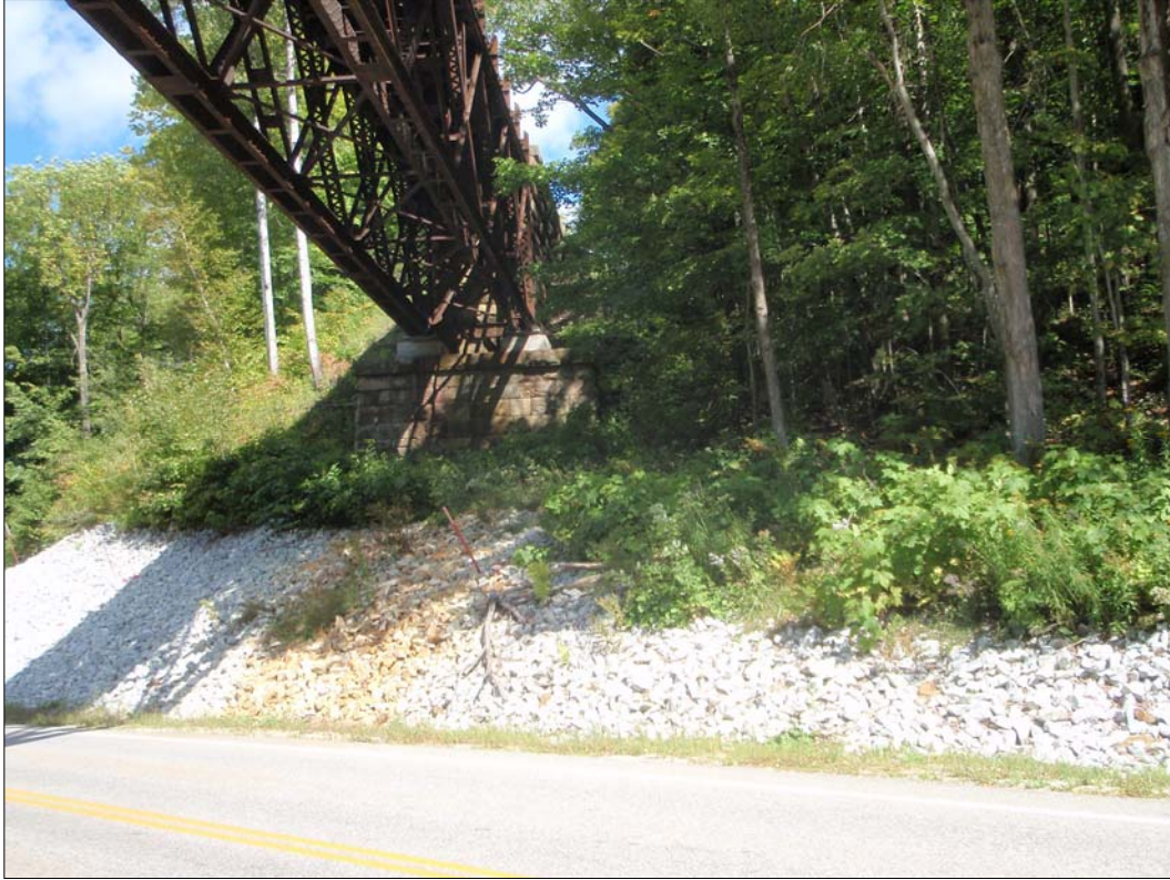
Photograph 5-87. Iron- trestle bridge over Freeman Brook at M.P. 137.5.
