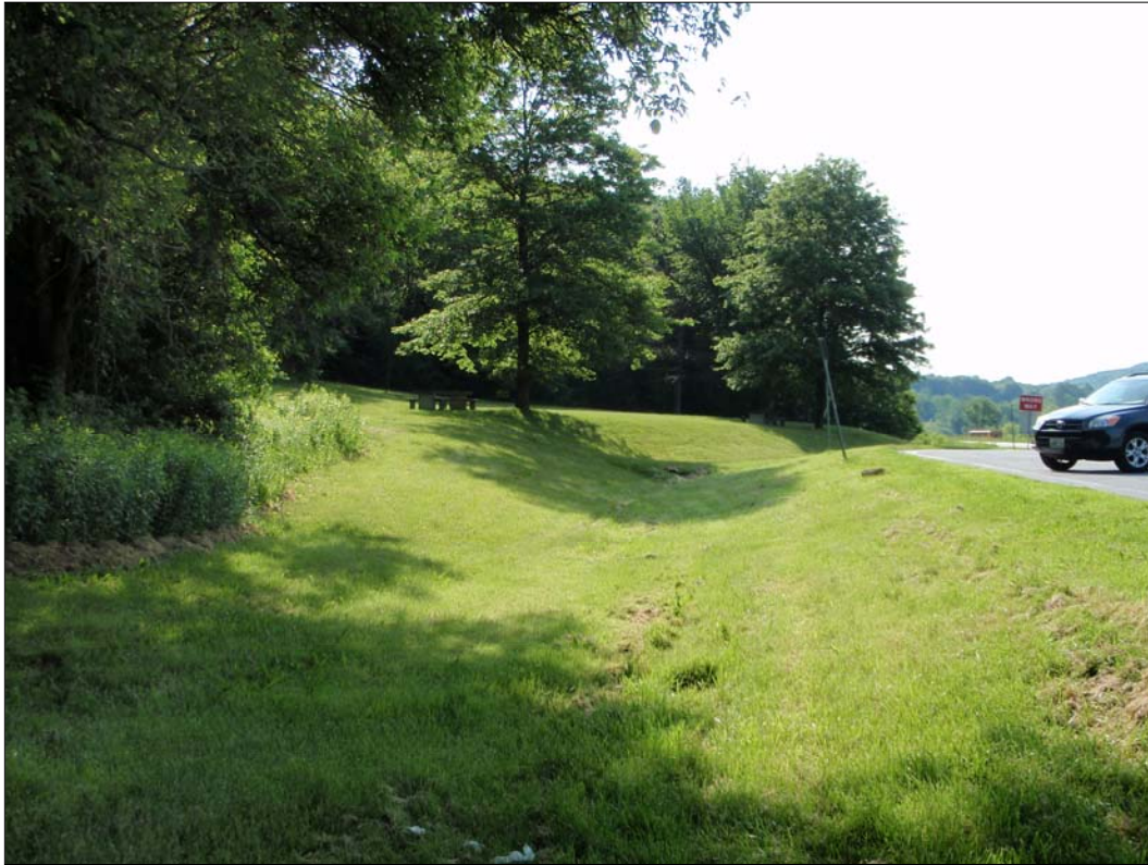
Photograph 5-61. Eastern two-thirds of Route 4 highway rest area at M.P. 120.2, view east.
