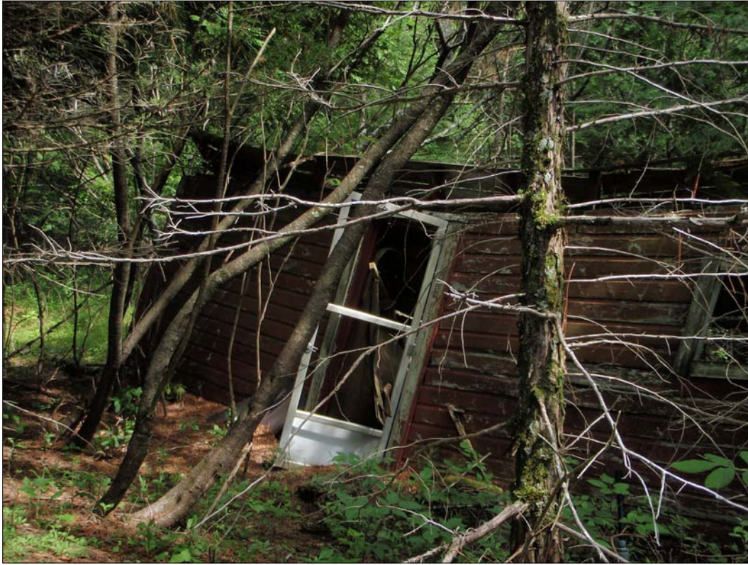
Photograph 5-13. Remain of modern hunting/fishing shack, Benson Parcel 2, view east.
