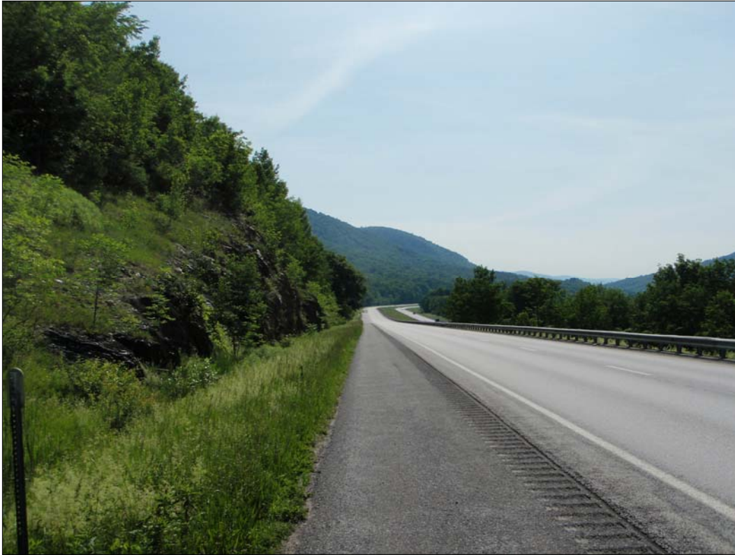
Photograph 5-57. View west from north side of Project at M.P. 119.9.
