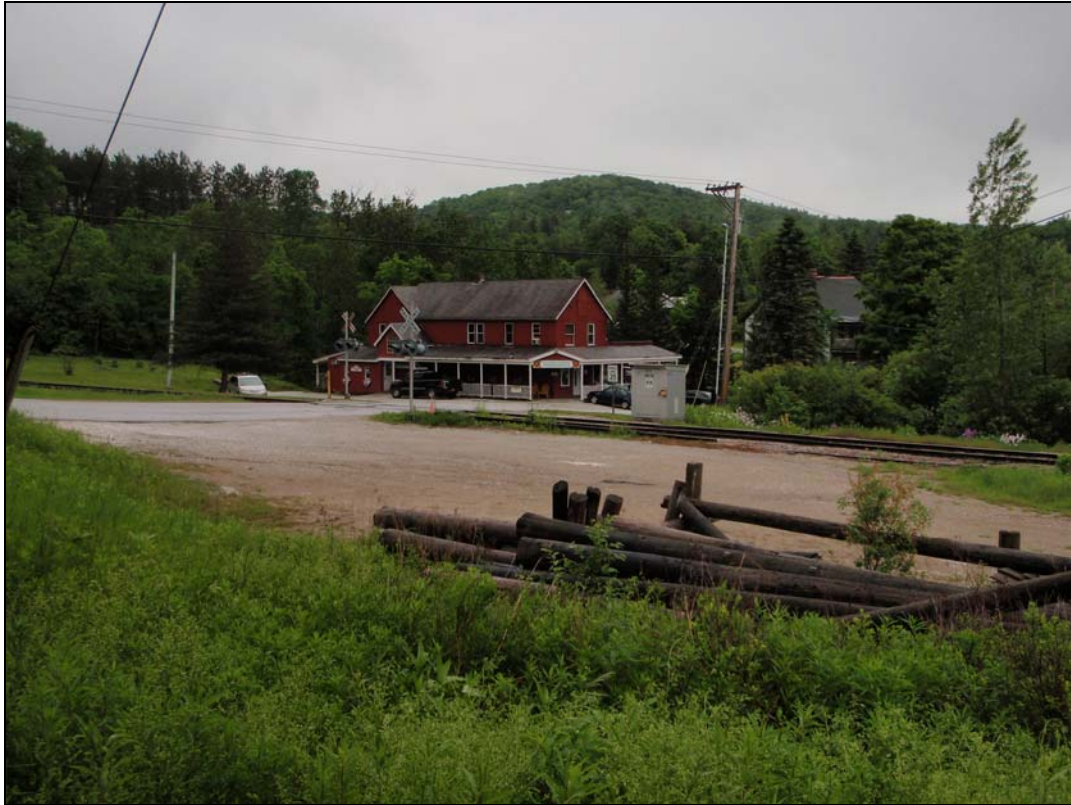
Photograph 5-95. View southwest toward Mount Holly railroad station from M.P. 140.9.
