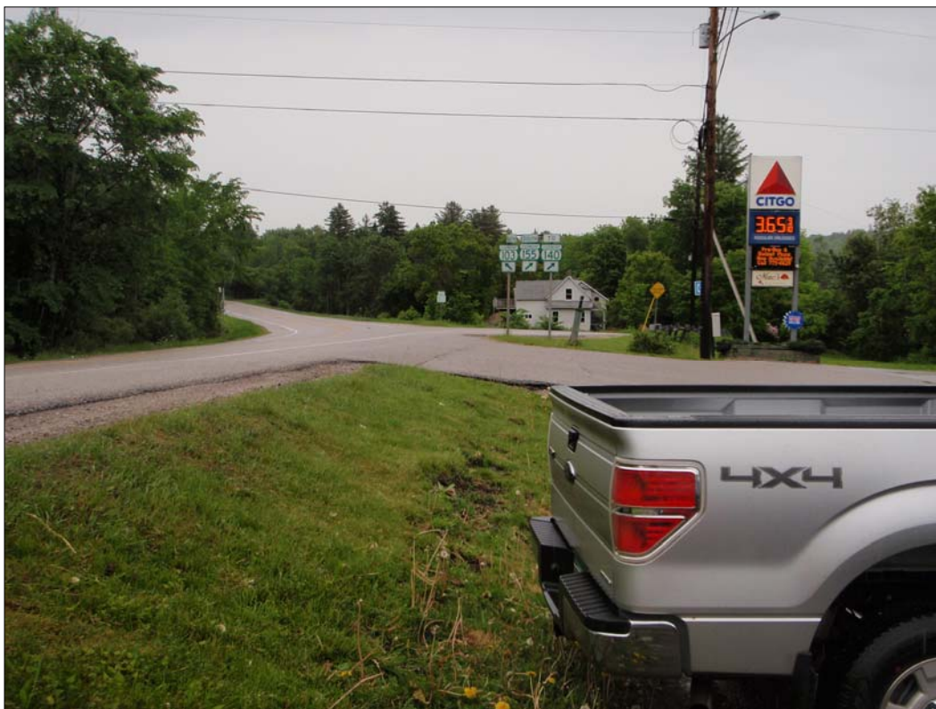
Photograph 5-90. View south from M.P. 138.2 showing typical road slope.
