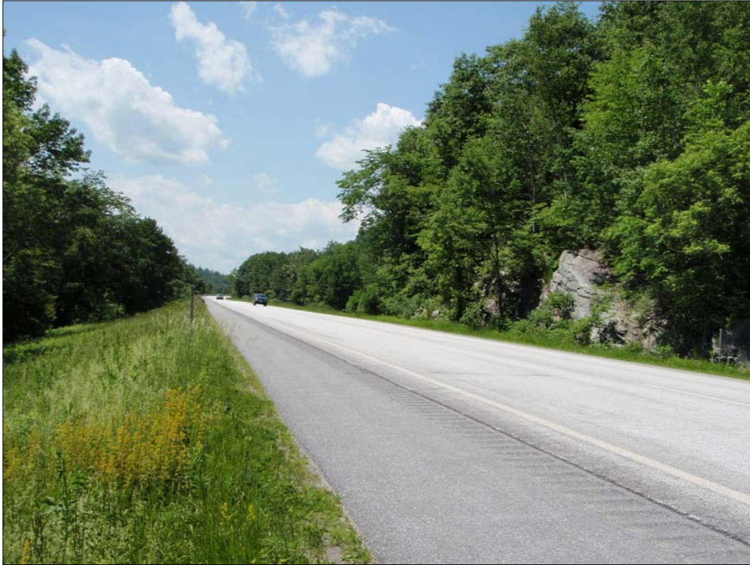
Photograph 5-49. View west along Route 4 eastbound from M.P. 117.95 showing steep road cut and exposed bedrock.
