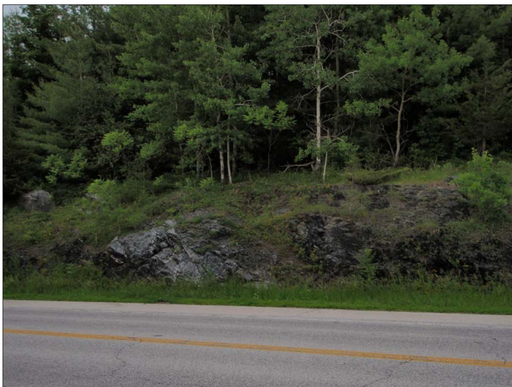
Photograph 5-33. Bedrock cut at M.P. 107.7, view east.
