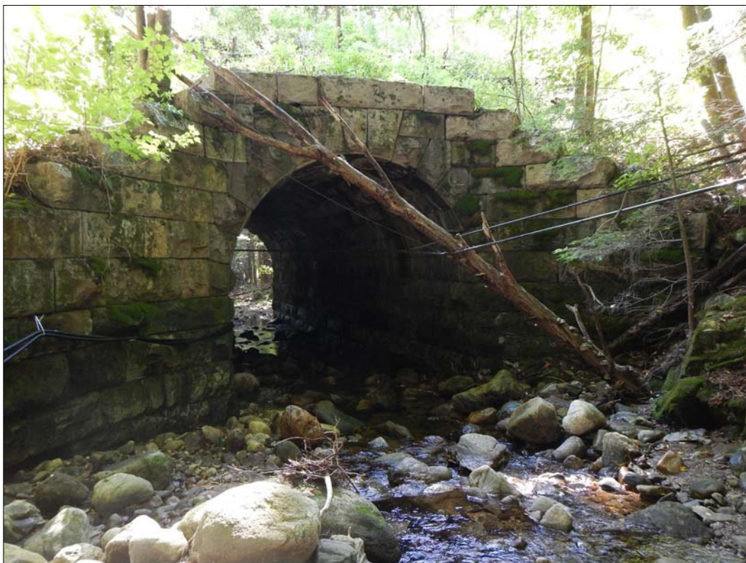
Photograph 5-84. Stone arch culvert at unnamed tributary to the Mill River at M.P. 134.6.
