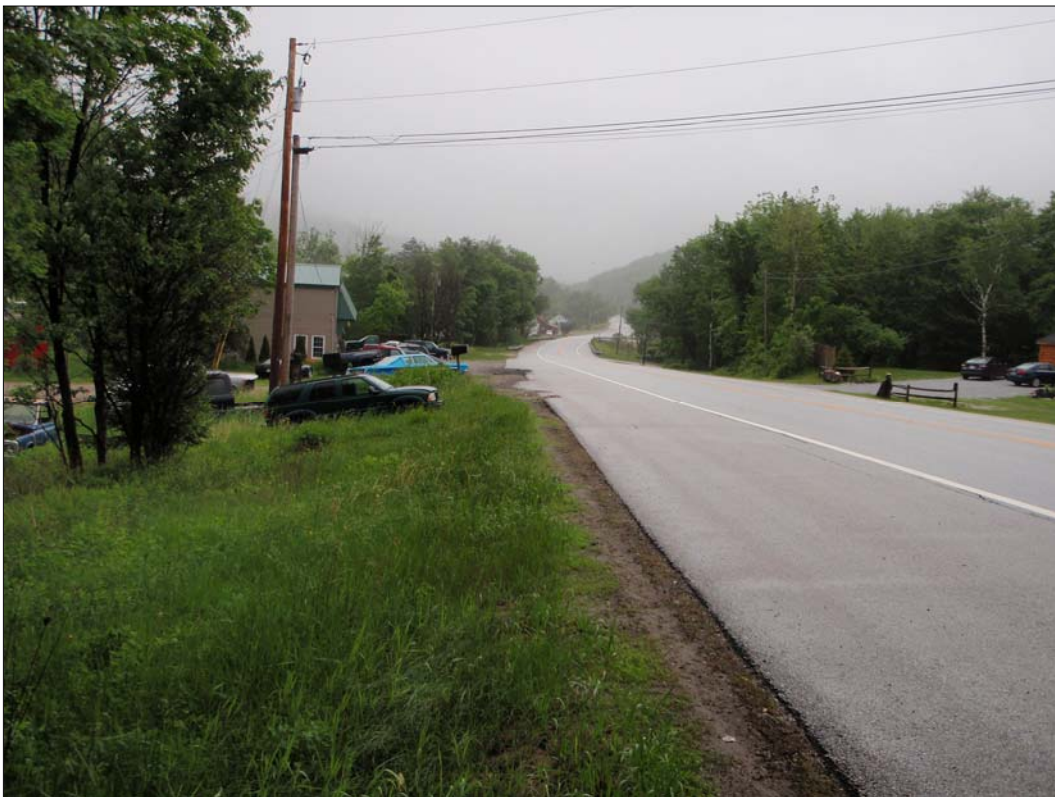
Photograph 5-99. View west along Route 103 from M.P. 145.1.
