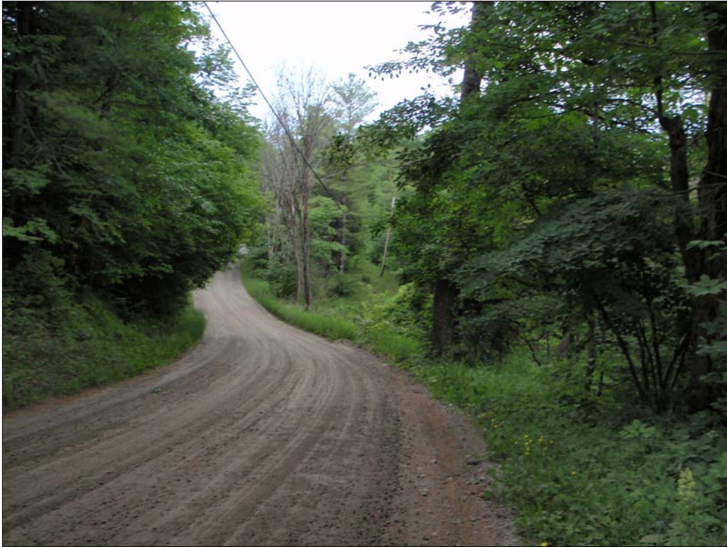
Photograph 5-22. M.P. 99.4–99.6 showing slope cut, view west.
