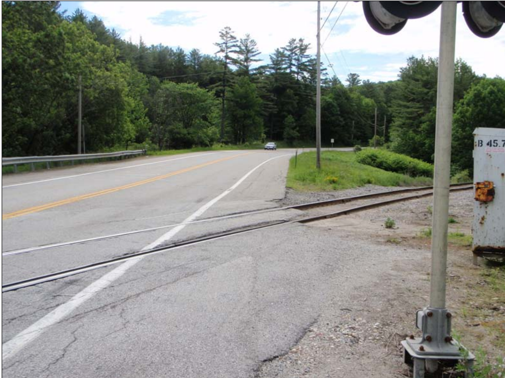
Photograph 5-79. View west from M.P. 132.7 showing cut landscape and railroad crossing.
