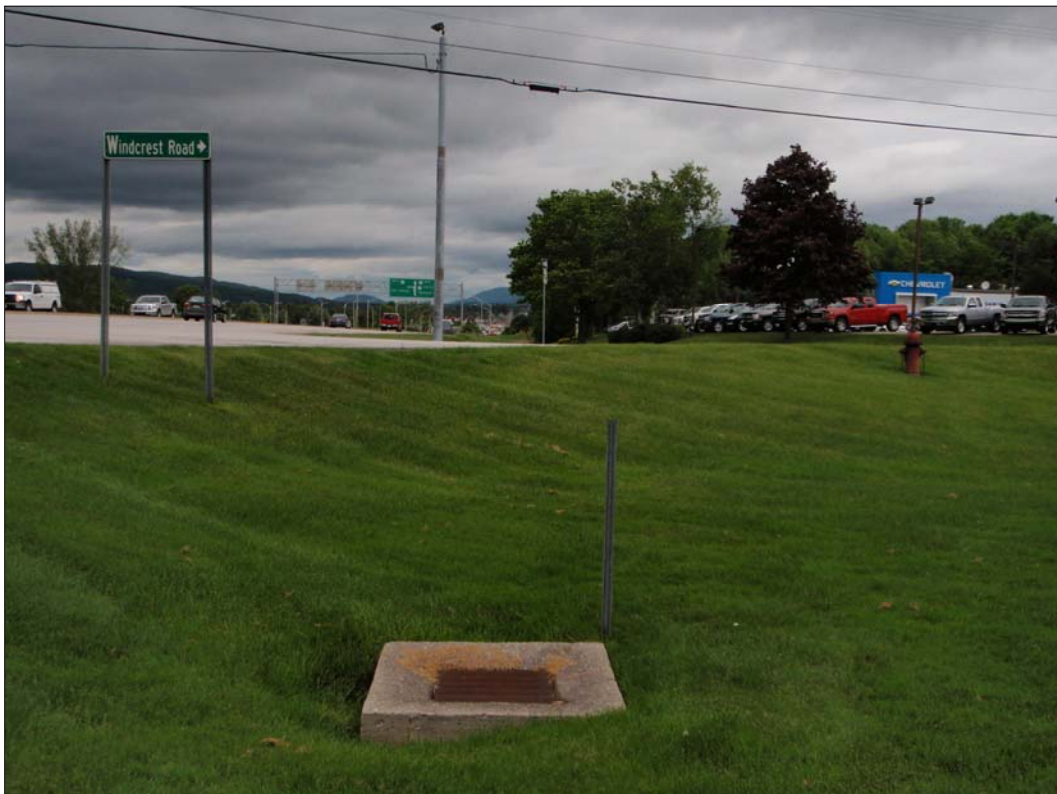
Photograph 5-70. View west from intersection of Middle Road and Route 7 at M.P. 128.05 showing drainage installations within south side of Project.
