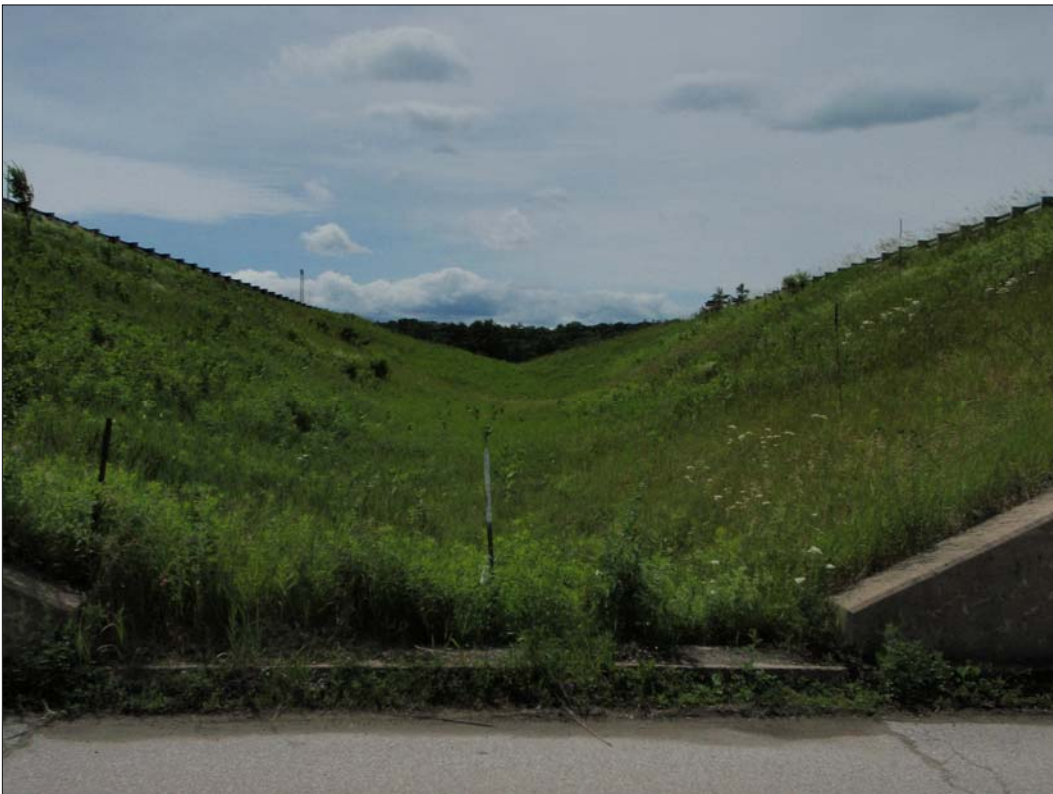
Photograph 5-41. View west from Airport Road between eastbound and southbound lanes of Route 4, M.P. 110.9.
