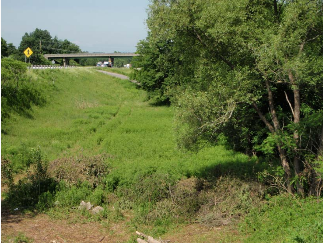
Photograph 5-51. General conditions within the Route 4/East Hubbardton Road interchange, view west.
