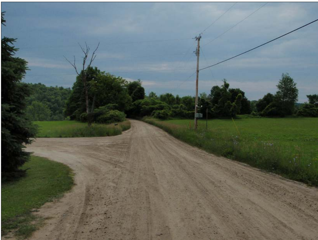
Photograph 5-20. Intersection of West Lake and Frazier Hill roads, M.P. 99.2–99.3, looking west.
