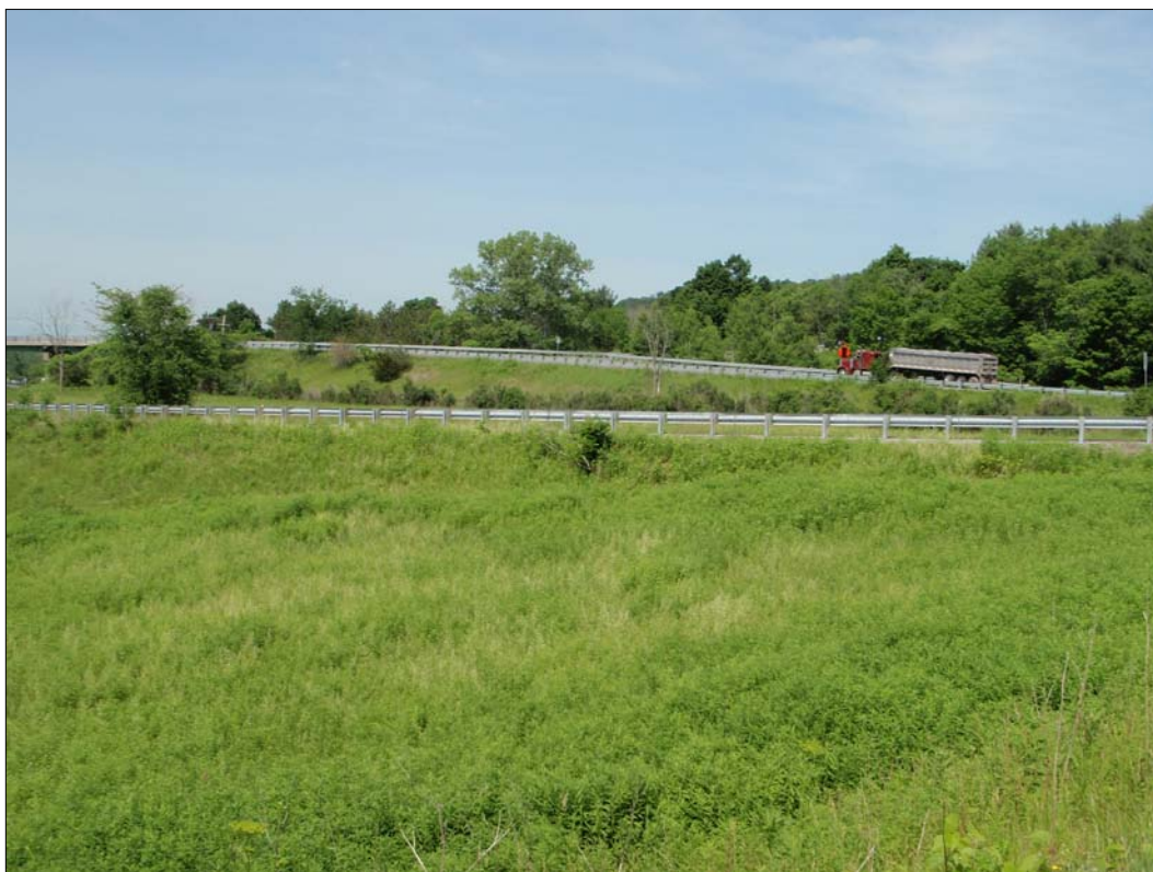
Photograph 5-53. Engineered slopes within the Route 4/East Hubbardton Road interchange, view west-northwest.
