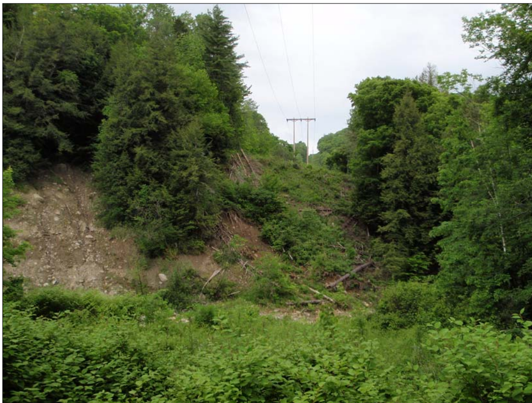
Photograph 5-88. Power line cut at M.P. 137.4, view northeast.
