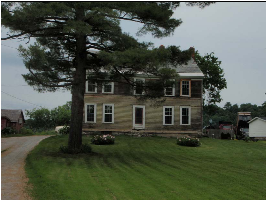
Photograph 5-29. A Briggs House, M.P. 104.9–105.0, view west.
