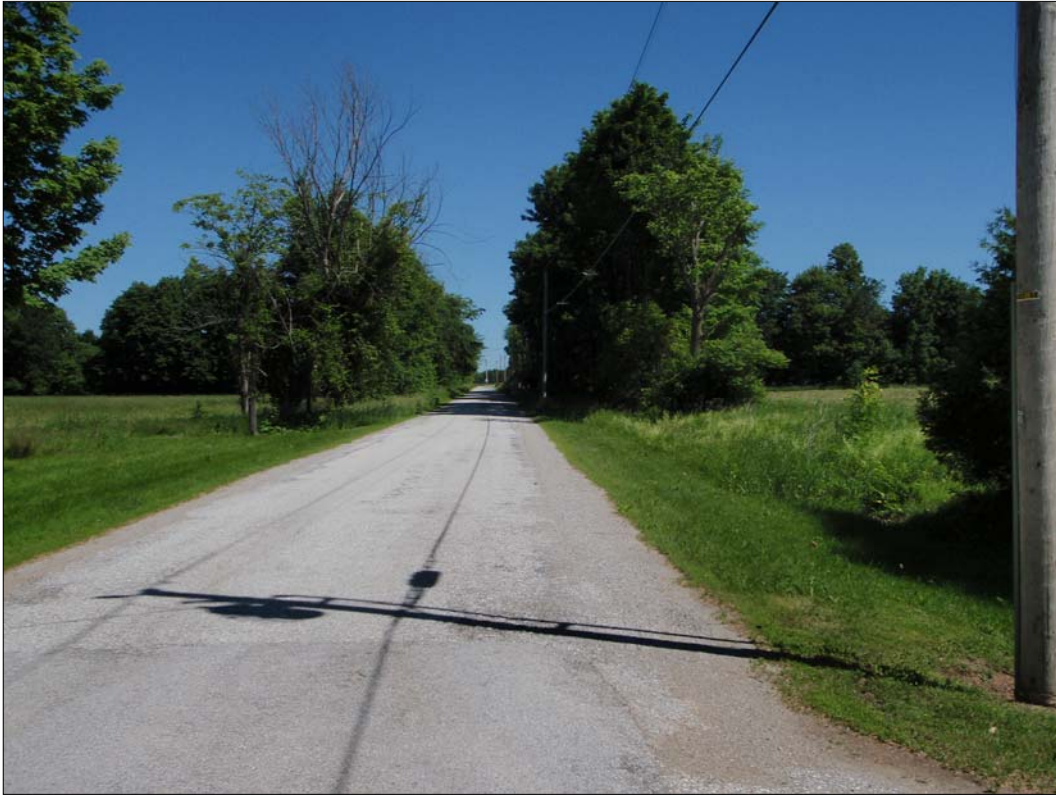
Photograph 5-1. Looking toward Line Road from the Florence Parcel (55 Bay Road), view north.
