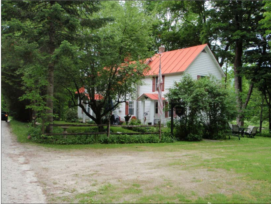
Photograph 5-107. Lakeside Saw Shop, M.P. 148.775.
