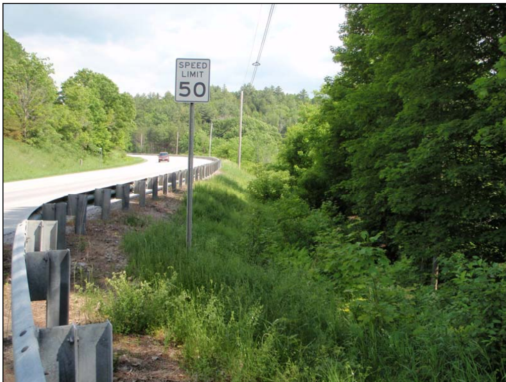
Photograph 5-80. ROW slope at M.P. 132.3, view southeast.
