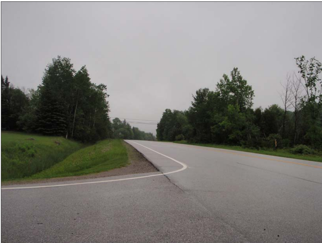
Photograph 5-97. View east along Route 103 from M.P. 143.7 showing drainage swale cut along the north side of the Project.
