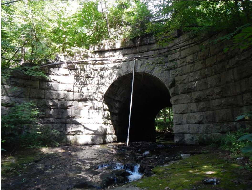
Photograph 5-85. Stone arch culvert at unnamed tributary to the Mill River west of Town Hill Road.
