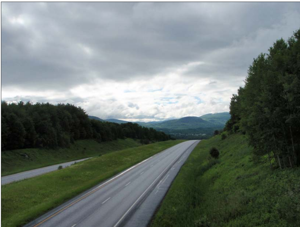
Photograph 5-66. View east from north side of Project showing east- and westbound lanes of Route 4, M.P. 125.7.
