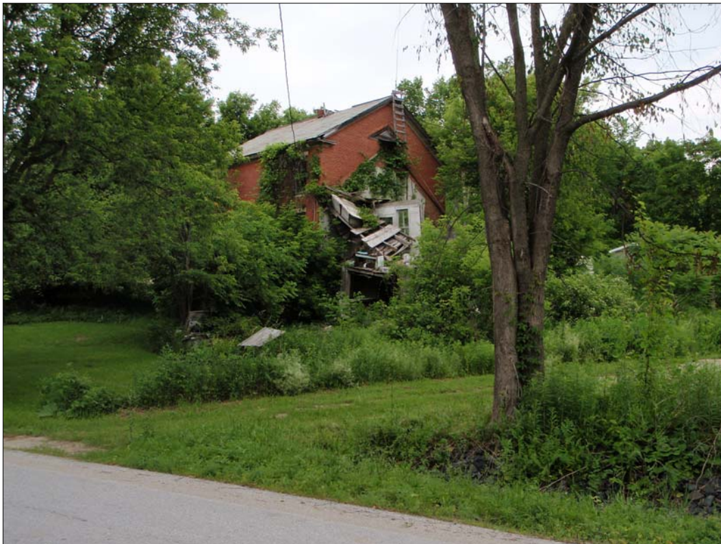
Photograph 5-25. View north toward the D.L. Osgood House from intersection of Stage and Hulett Hill roads.
