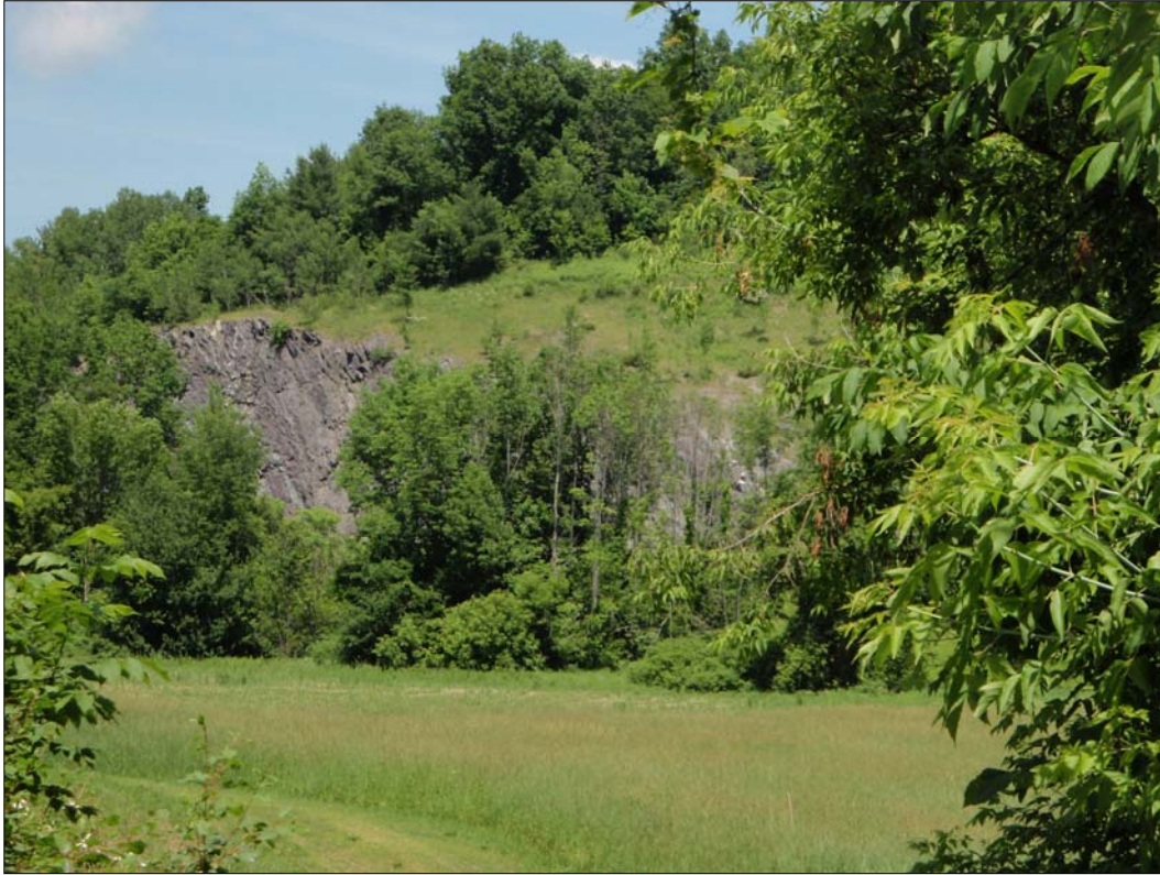
Photograph 5-54. Blasted bedrock in southern portion of Route 4/East Hubbardton Road interchange, view north.
