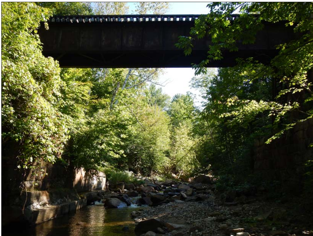
Photograph 5-86. Rail deck at Freeman Brook.
