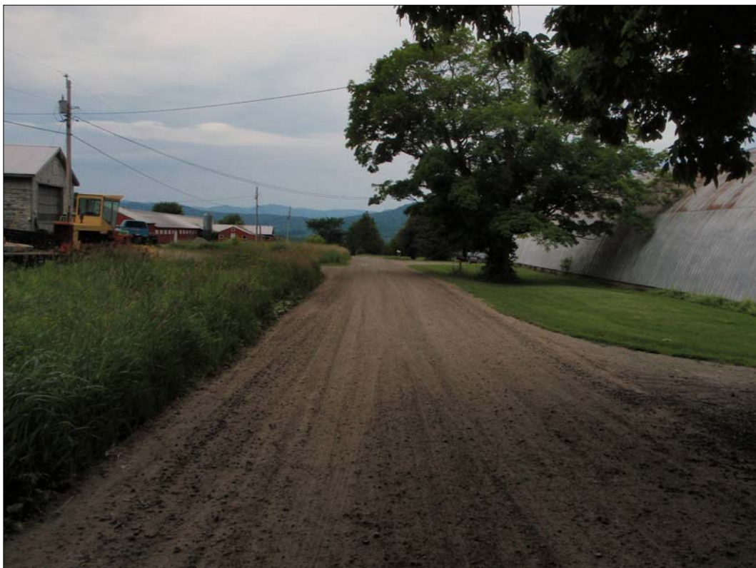
Photograph 5-17. M.P. 98.96 looking west down West Lake Road.
